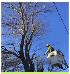
A primary cause of power outages is trees contacting power lines. CCECA makes every effort to provide you with safe and reliable electric service.
