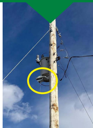
You may notice this device on various poles in our service territory. This device helps boost the signal from our meters back to our office.
